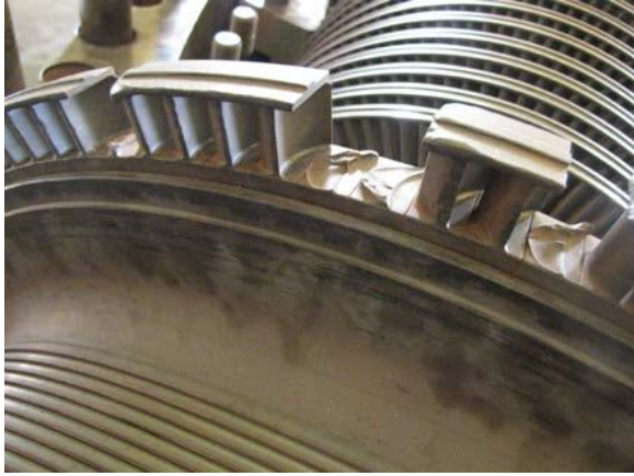
Figure 12. Hp broken blades (Detail shot)
