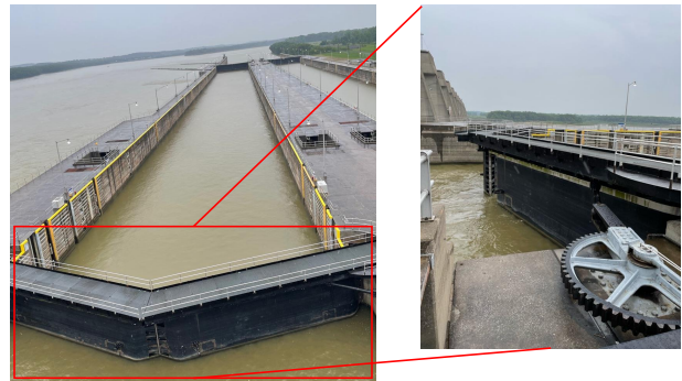
Figure 1. Miter gates in inland waterway lock systems
