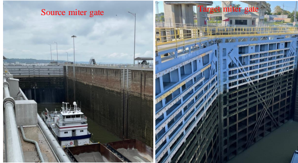
Figure 7. Illustration of source and target miter gates on a river.
