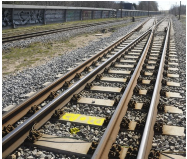
(a) Overview of the turnout in proximity of Tommerup station
