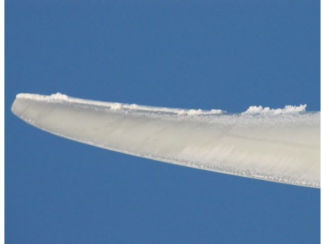
Figure 2 Icing on Wind Turbine Blade
