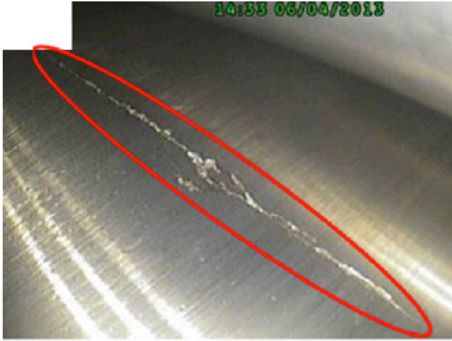
Figure 3 Damaged High-Speed Bearing, HI 1.1
