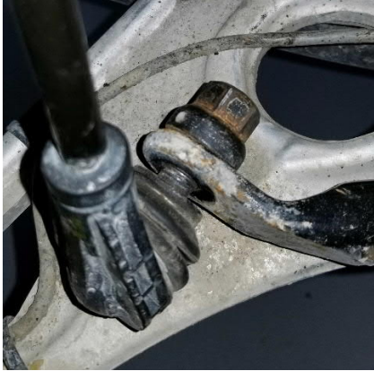
Figure 1 Loose end link of stabilizer bar on the vehicle
