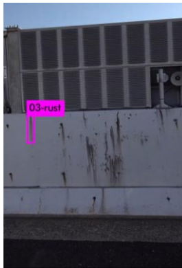
Figure 7. Object extraction from rust juice by deep learning of wall balustrade
