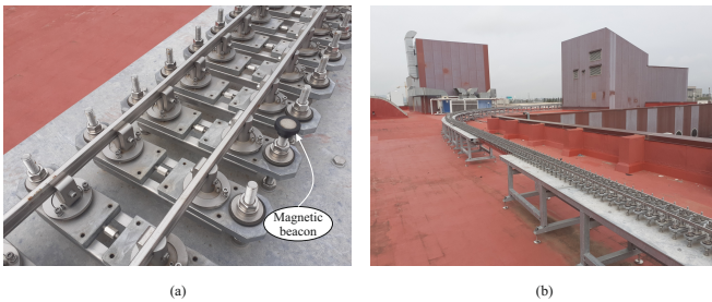
Figure 2. (a) Track sleepers. (b) Track overall view
