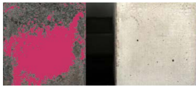
(b) Efflorescence from original image
