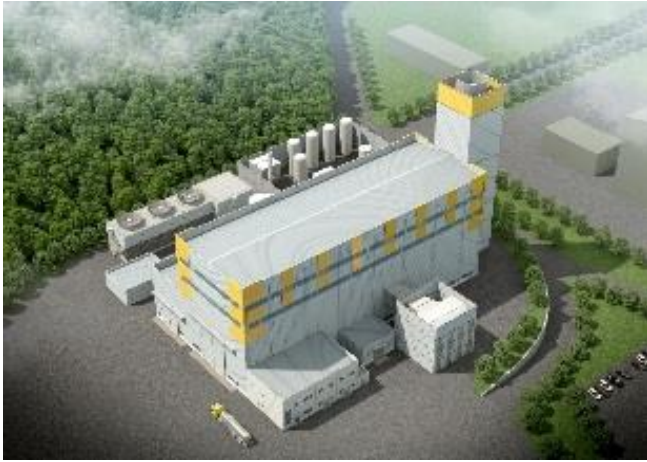
Figure 9. DHI FSFL test facility
